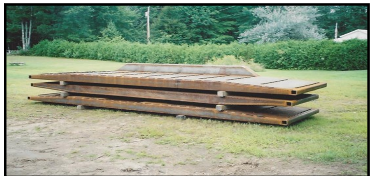
Example of an all-Steel Skidder Bridge
