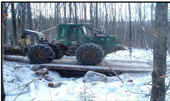
Wooden Skidder Bridge
