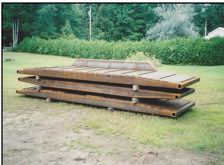
Example of an all-Steel Skidder Bridge
