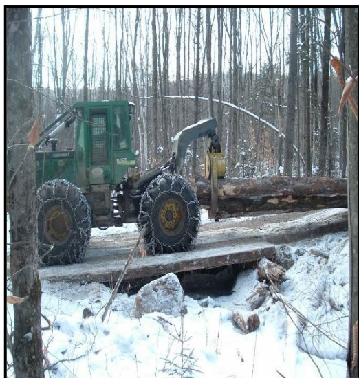
Wooden Skidder Bridge
